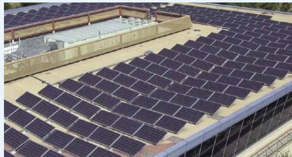
Figure 4 - Solar Panel Inspection
